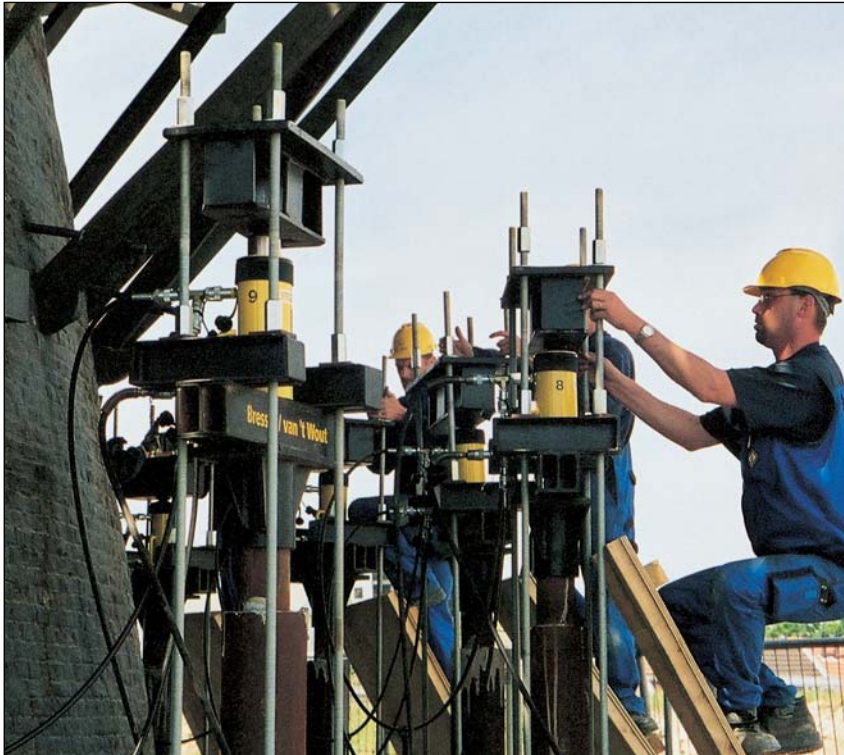
▼ Stage-Lift System used for lifting a windmill
